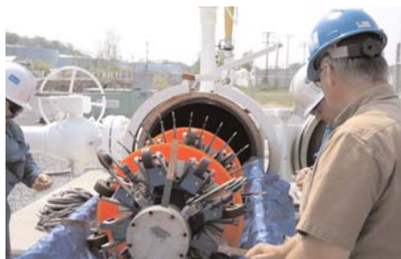
Insertion of pig into launcher
