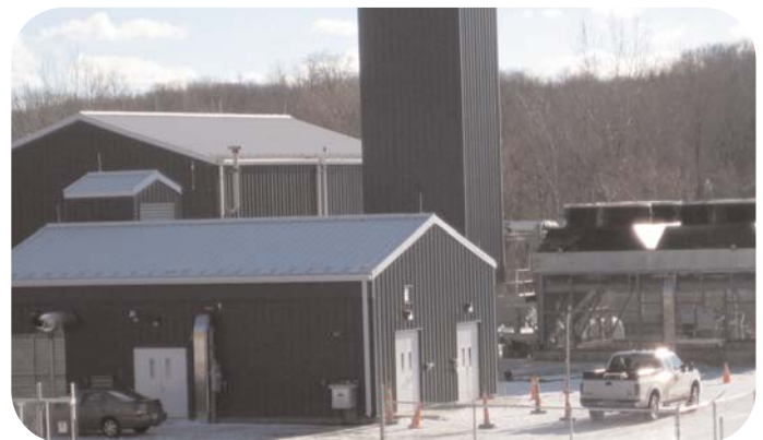
Brookfield, CT: The 7,700 hp transfer compressor station began operations November 1, 2008.
