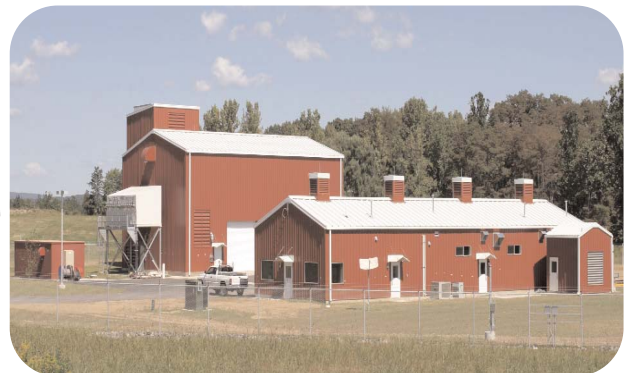
Dover Compressor Station
