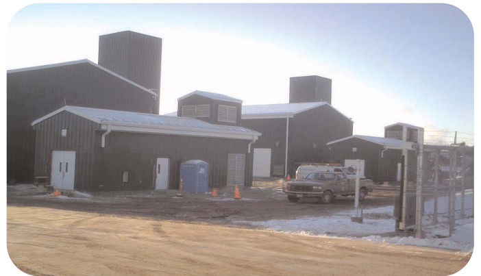
Milford, CT: New compressor station, housing twin 10,300 hp turbines, began operations January 14, 2009.
