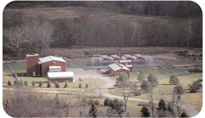
Dover, NY: A picturesque view of the entire facility shows the new gas coolers.
