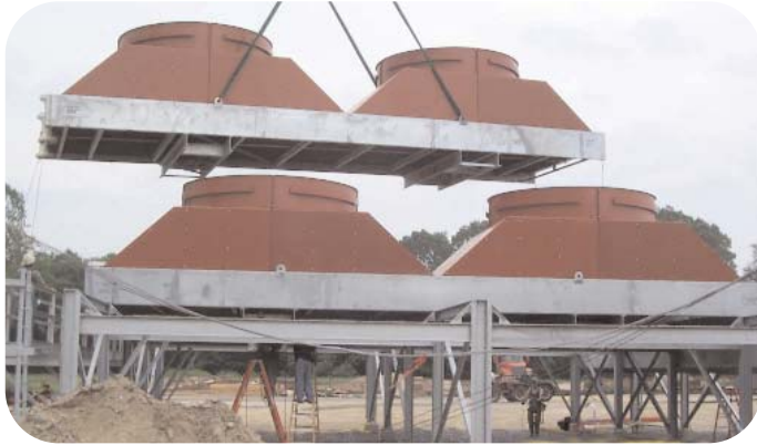
Dover, NY: Gas cooling fans are lifted into place.
