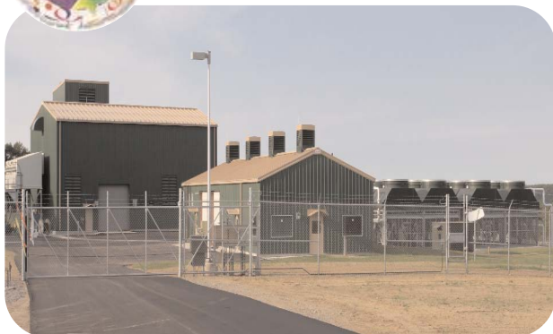
Boonville Compressor Station
