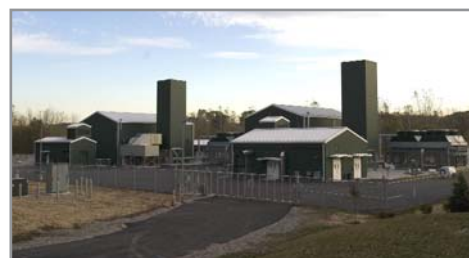
Phase III: Addition of a second compressor unit (left) at Brookfield Compressor Station
